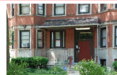
Tabitha House Residential Womens Treatment Facility
